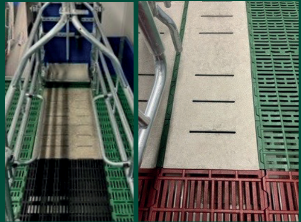
Concrete slats in combination with cast iron slats and plastic slats.
